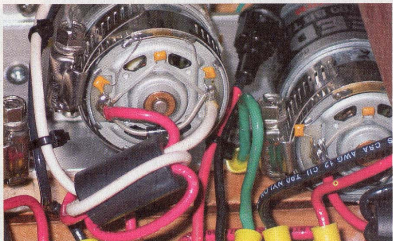
Motors are the main source of glitch-inducing RFI. To fight glitching, this motor is well set up with capacitors, ferrite beads and a transient suppressor.
